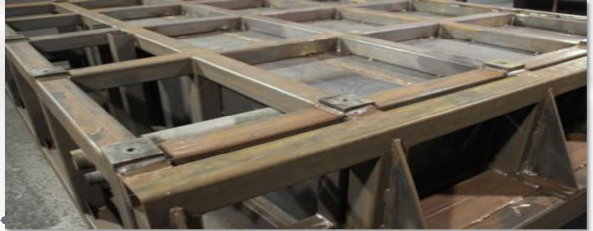
Before sand blasting
